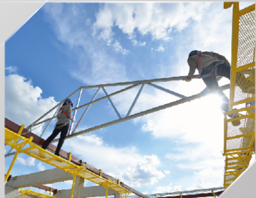
The sky walker specifically designed for SCG is used for work safety.
