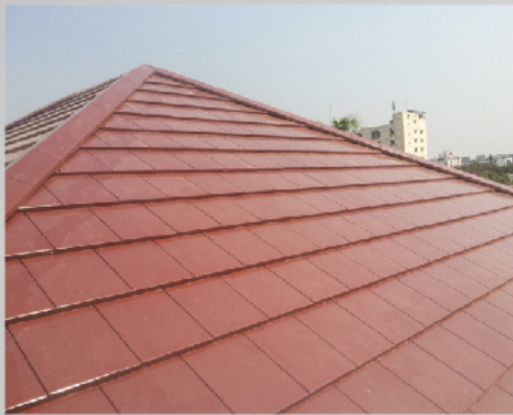
Tightly sealed roof sheets with no leaks
